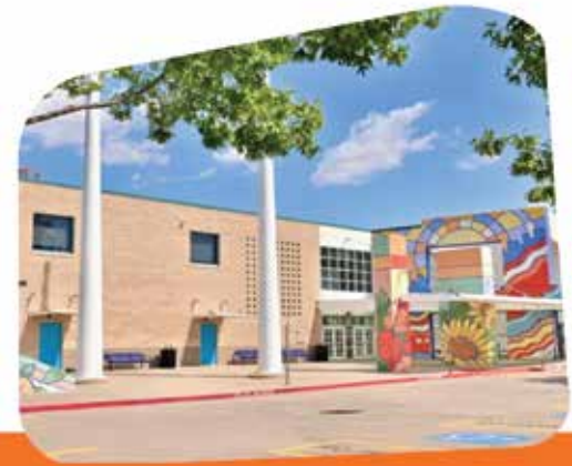
Denver Harbor Multi-Service Center
